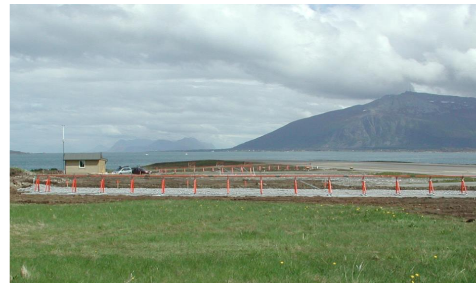
Our Model 105 End-Fire GS Antenna System commissioned in Vigra, Norway
